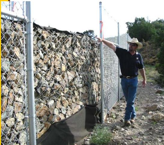
*NMDOT Project Manager Ted Barela shows that the drop on the outside of the escape ramp will keep wildlife from going back up onto I-40.*
