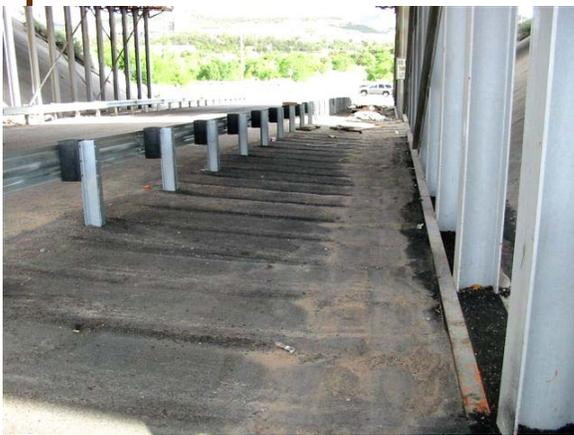
The widened and baffled shoulder will trap sediment for a better substrate at the Public School Road underpass.
