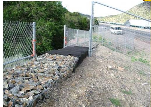
*Escape ramps direct animals running along the fence up the slope to the opening.*
